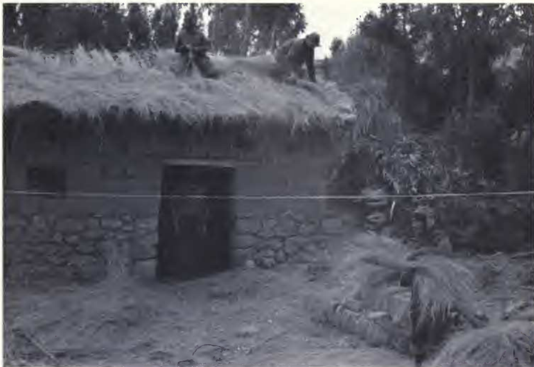
FIG. 8. An ayni group works together to construct a new house (photo CCTC).
